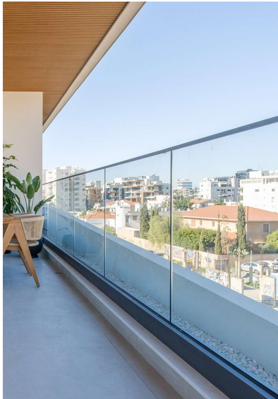
GLASS BALUSTRADES MU585 (or equivalent) (RAL7021 or equivalent) Height : 1.1m
